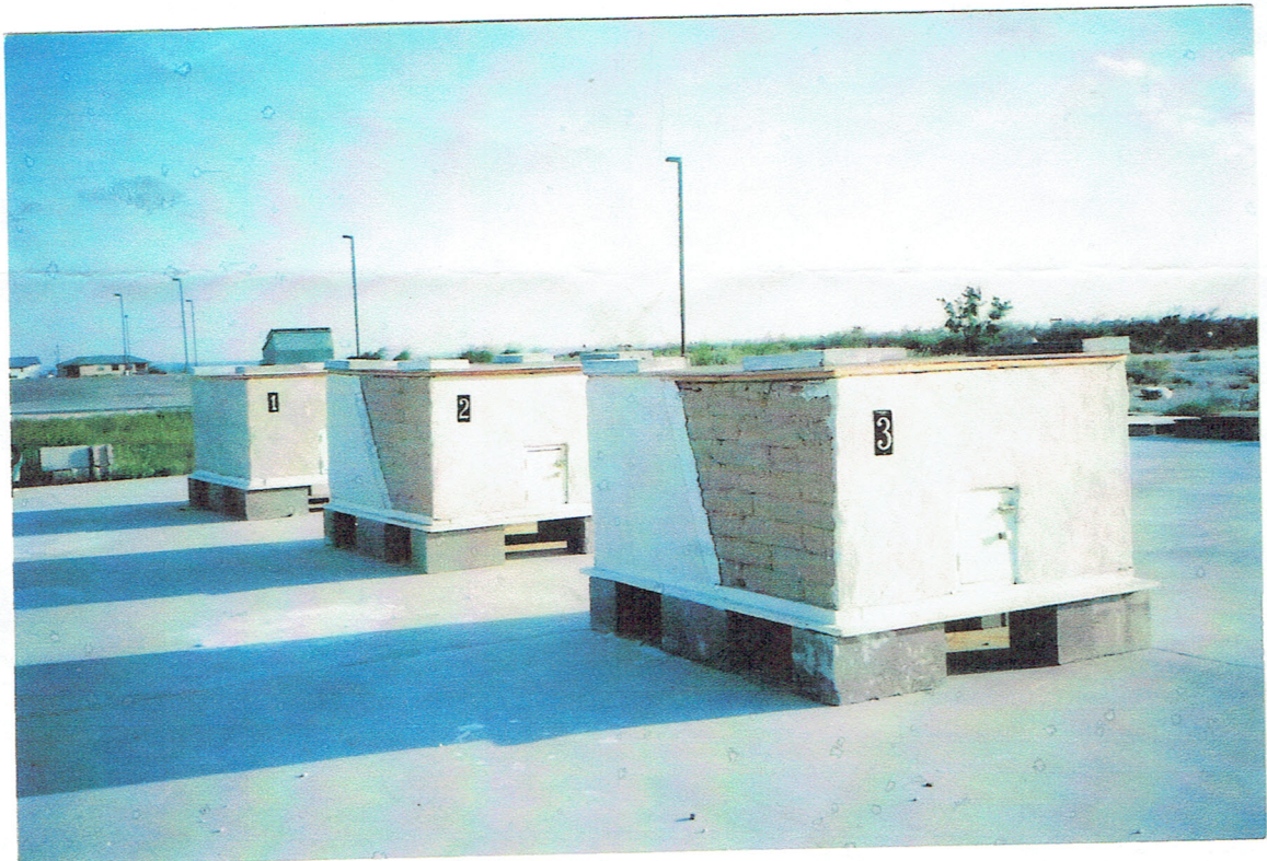
Three modules facing due north. From left to right: #1 concrete block, #2 adobe and #3 compressed earth block. The partial render on the two earthen modules allows exposure to the wall for taking moisture data and to illustrate a two-coated lime render. Modules rest on 8-inch concrete blocks.
